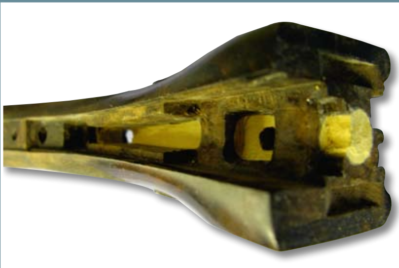
THE DOWEL INSERTED AND HEADED UP FOR THE ACTION
